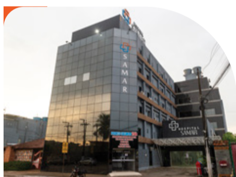
Hospital Samar Centro
